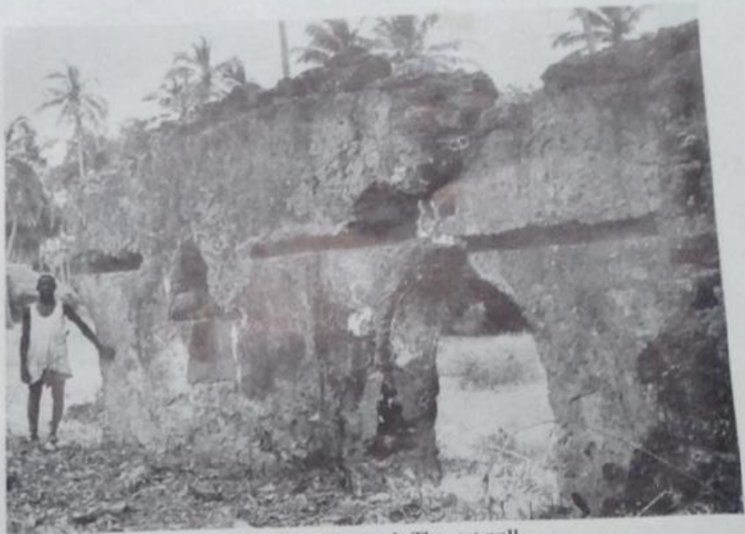
Plate IA. Mosque I: The east wall.
