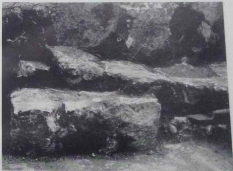
Plate VA. Pilaster on west side of Mosque III, covered by floor \alpha . The trowel is inserted on floor \beta and floor \gamma is in the foreground.
